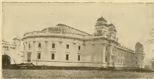
ORIENTAL EXHIBIT BUILDING.
